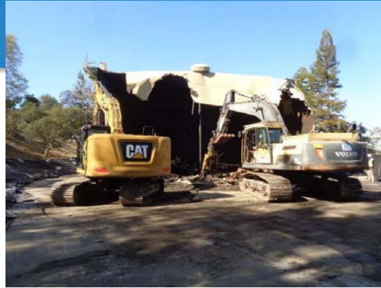
SJW Montego Station – Welded Steel Tank Demolition
