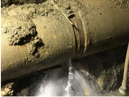
Leak on a 42-in Steel Pipe
