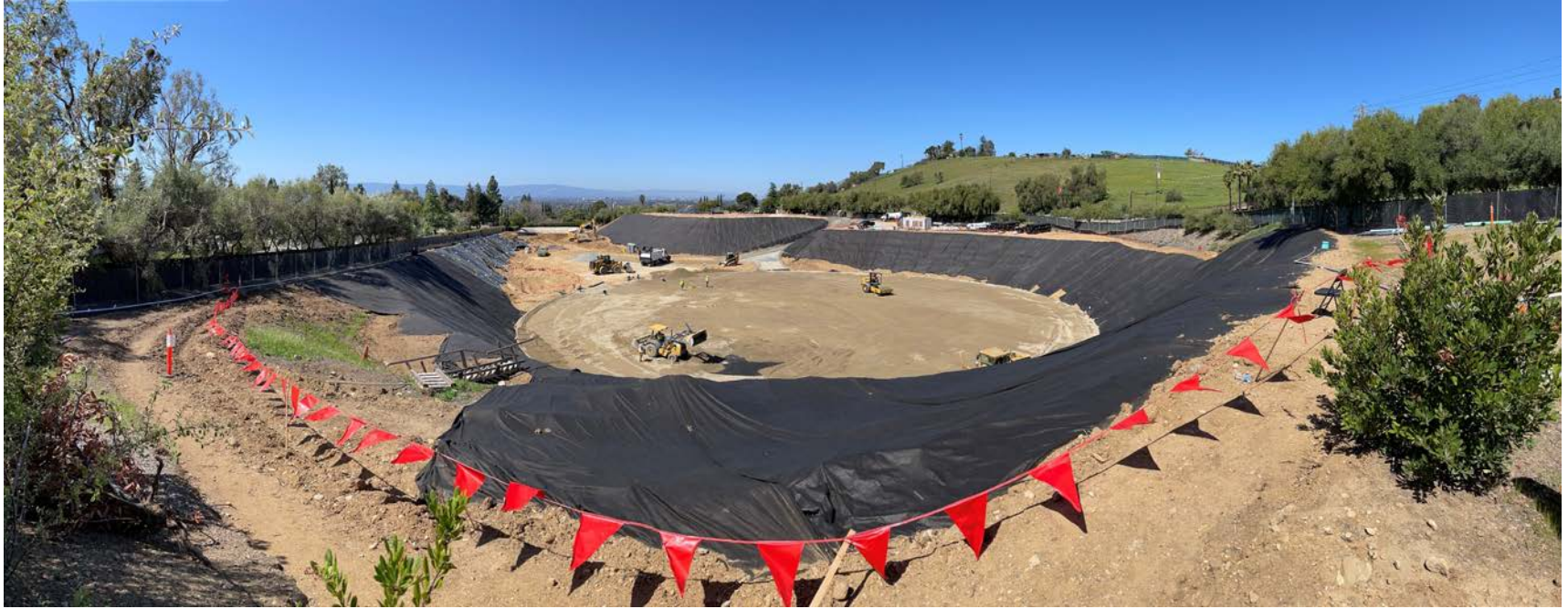
Construction Progress Photo Taken in March 2021 After Demolition of the Existing Earthen Embankment Reservoir and Phase 1 Grading Activities for Tank 1 Construction
