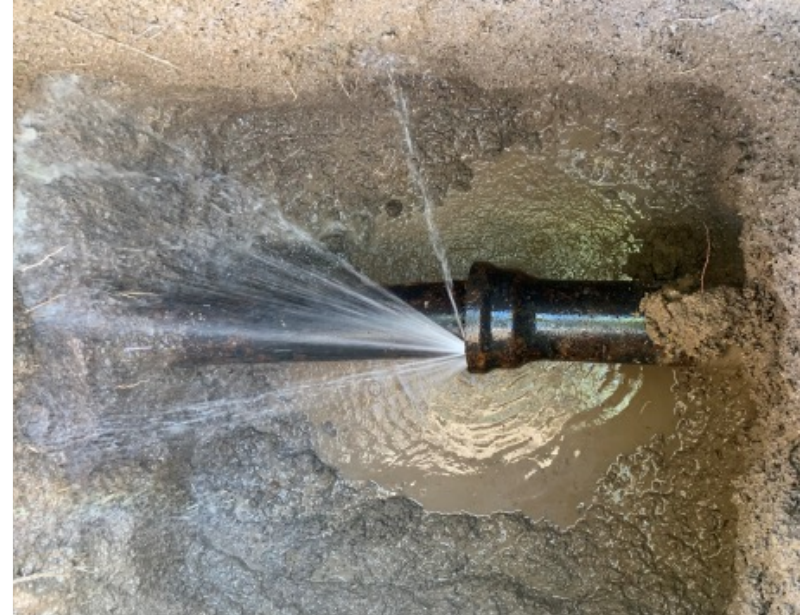
Leak at joint
